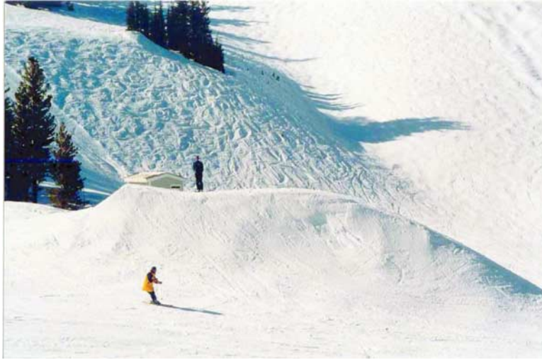
FIG. 1—Typical large terrain-park tabletop jump. Jumper approaches from takeoff ramp on the left, is airborne over the roughly horizontal tabletop, and lands on the nearly constant down-slope to the right.
